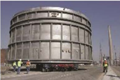
Figure 3 Example of a 2205 stainless steel scrubber tank
