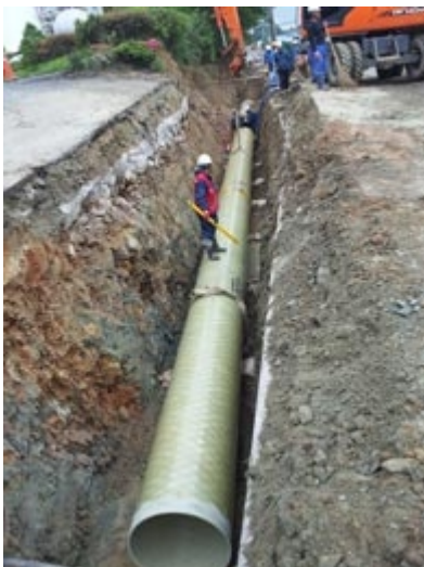
Figure 1 Installation of Advantex® Glass reinforced FRP pipe in South Korea
