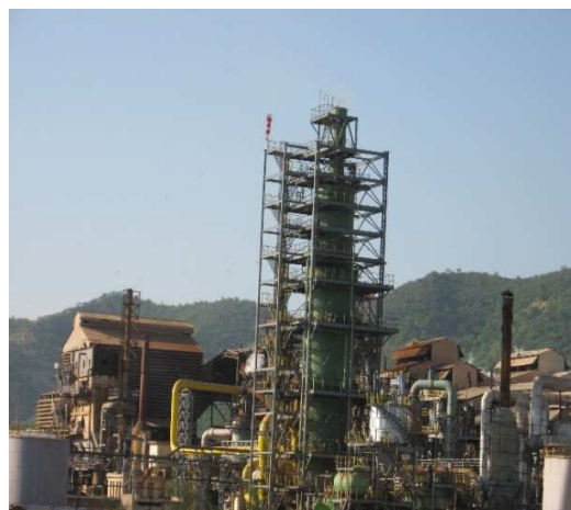
Figure 2 FRP Scrubber being installed on location in Saudi Arabia
