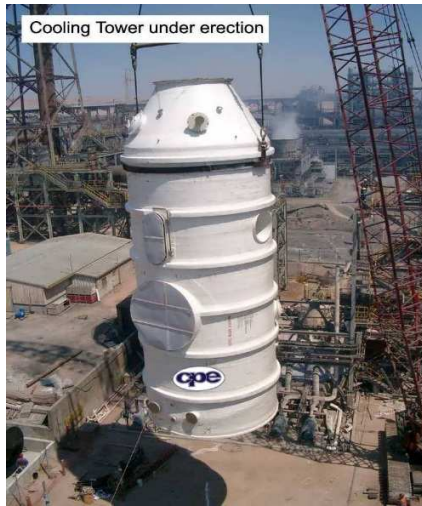
Figure 3 FRP Cooling tower being erected
